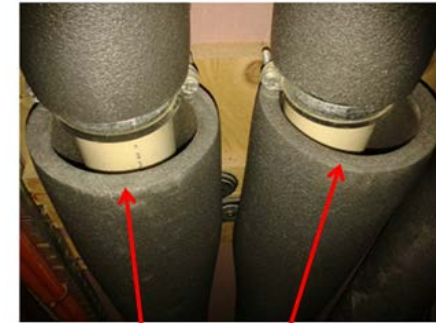
Loosely fitted insulation which allows great inefficiency.
