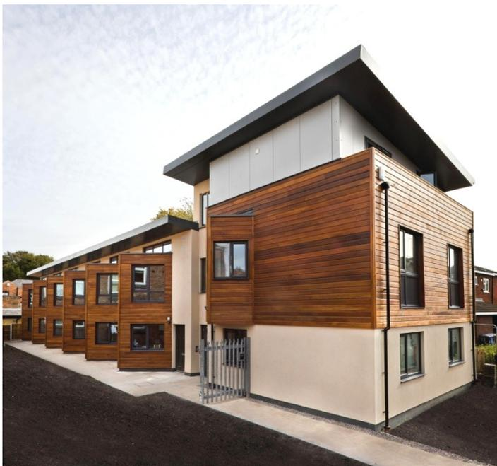
**Fabric** Highly insulated ICF (Integrated Concrete Forms) walls and steel roof, combined with triple glazed windows and high airtightness performance result in a highly efficient fabric.
