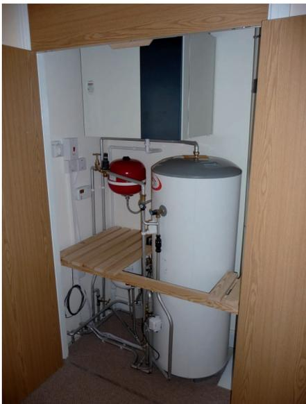
Good practice: MVHR unit (above cylinder) in easily accessible position and within the heated envelope of the home
