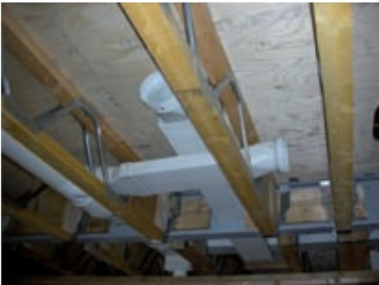
Design innovation allows space-saving inclusion of MVHR ducting and ease of installation.
